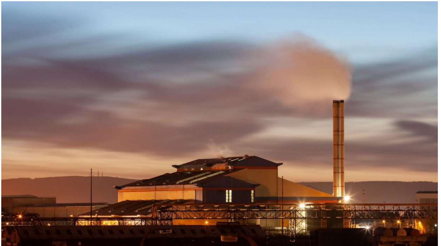
A waste-to-energy incinerator at Haverton Hill near Middlesbrough, England. ISLANDSTOCK / ALAMY STOCK PHOTO
