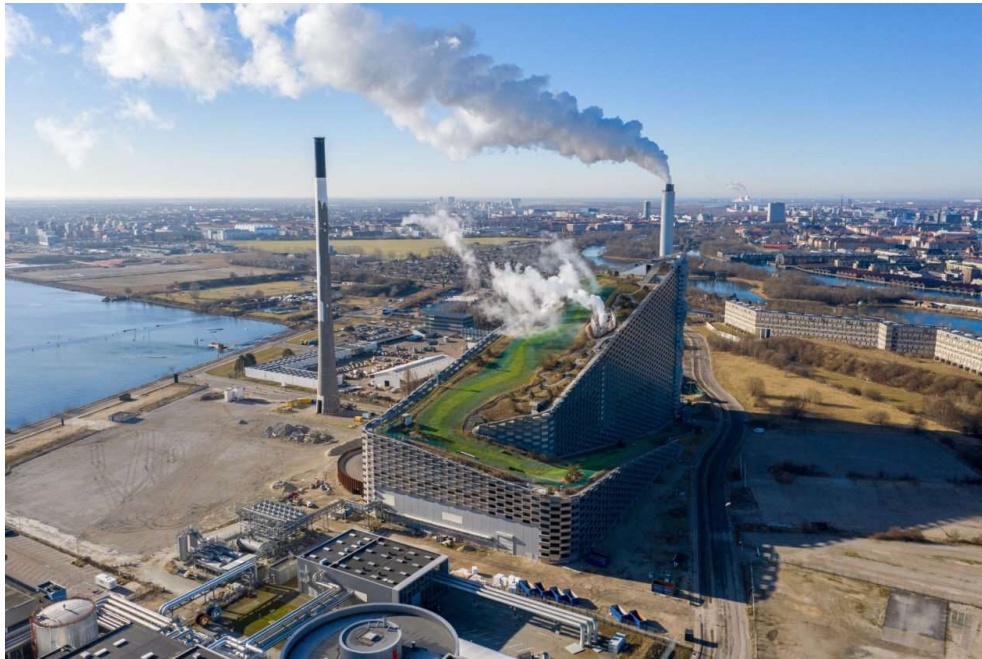
The Amager Bakke waste incinerator in Copenhagen, Denmark has a ski slope on its roof. OLIVER FÖRSTNER / ALAMY STOCK PHOTO
