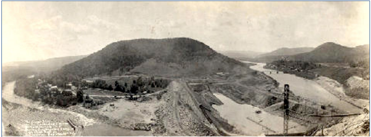
Conklingville Dam under construction
