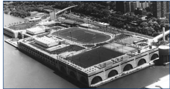
New York City's North River Treatment Plant
