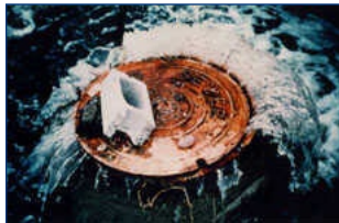
Rain can overload sewers
